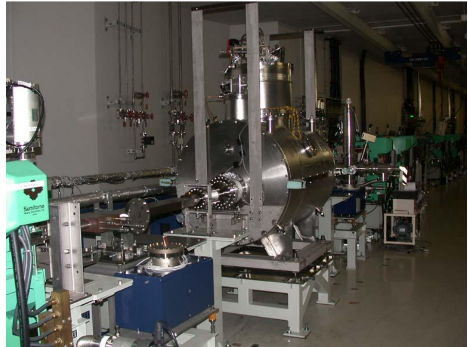
10 Tesla WLS installed on SPring-8
